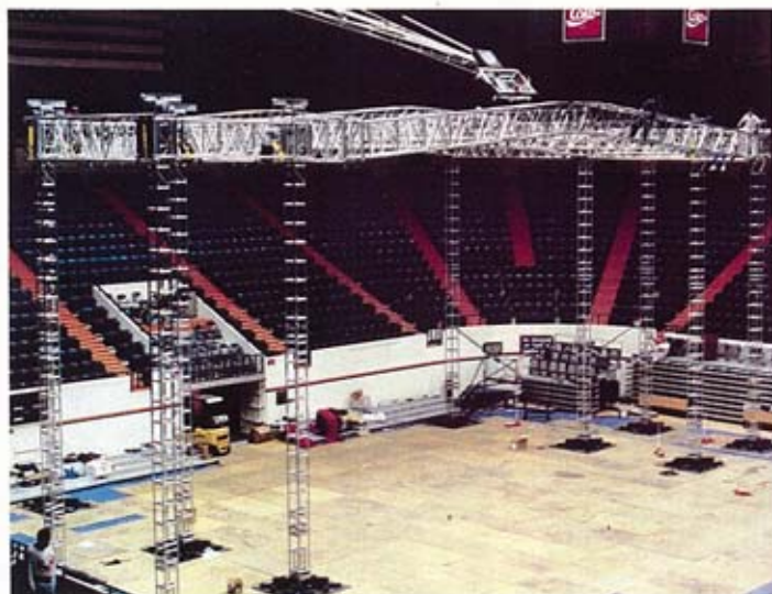
A structure for Clemson University, South Carolina . . .
